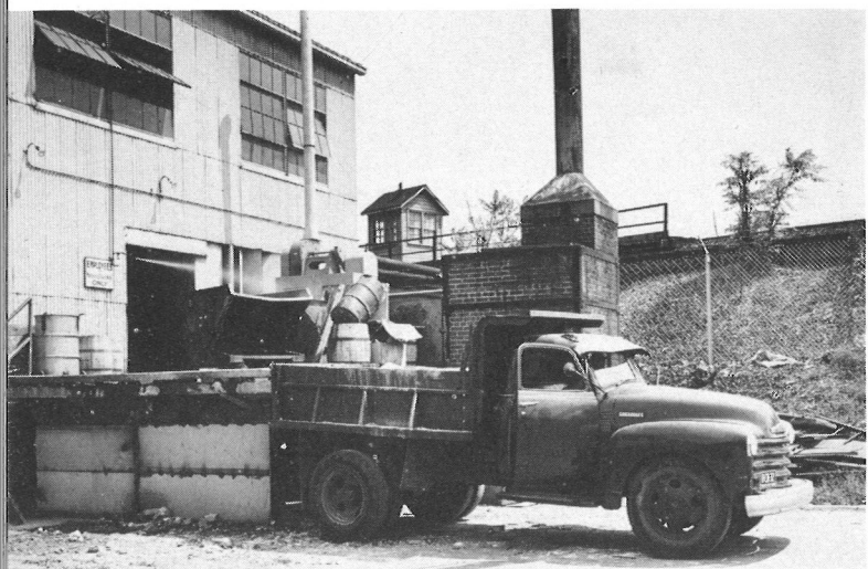
Rubble carts are sprayed outside while awaiting dumping. Stack at left is part of dust collector for masonry saw.
